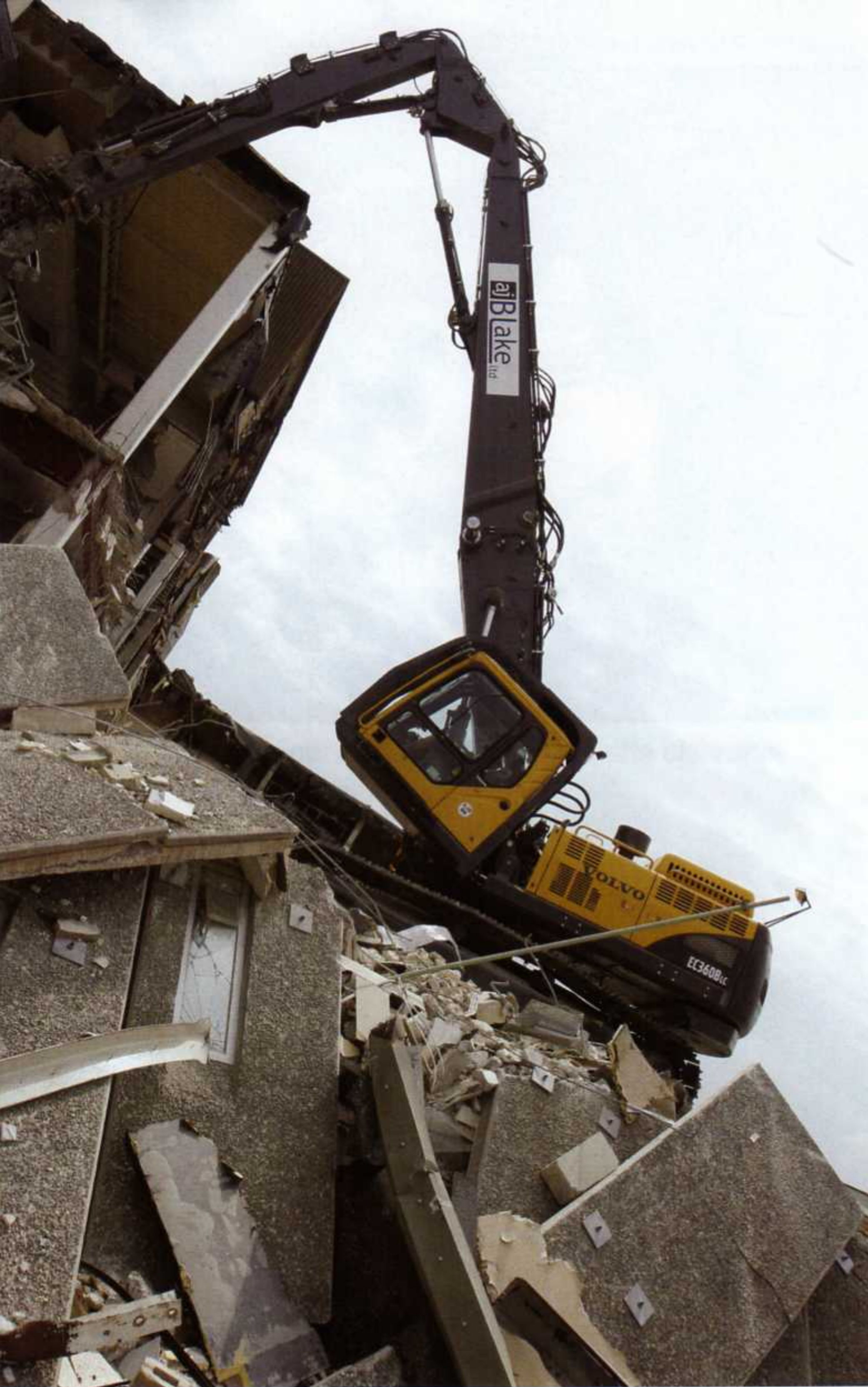
Left: The Volvo rig features a tilting, armoured and caged cab, an additional counterweight in addition to belly and track guards.
